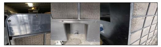
4. Use a water supply hose to manually fill the reservoir to the full level on the level indicator panel located at the rear of the unit below the air inlet panels, or if overfilled drain off the excess water to the correct full levelFill water tank to recommended level and test unit for operation.
